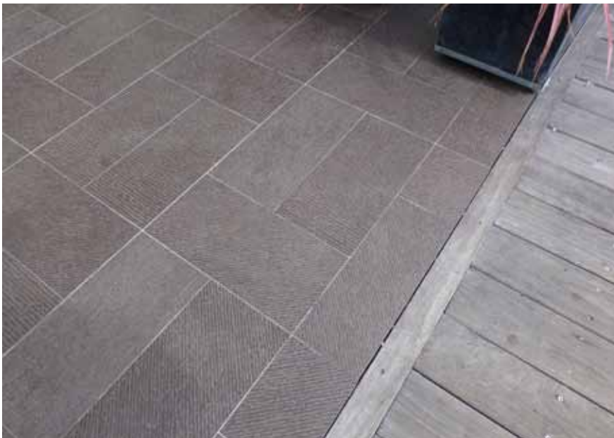
ABOVE: Paving laid in 2011 in Harris Street, Pyrmont
